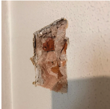
Figure 10 Wall between Living room and Dining room makeup near external wall.
