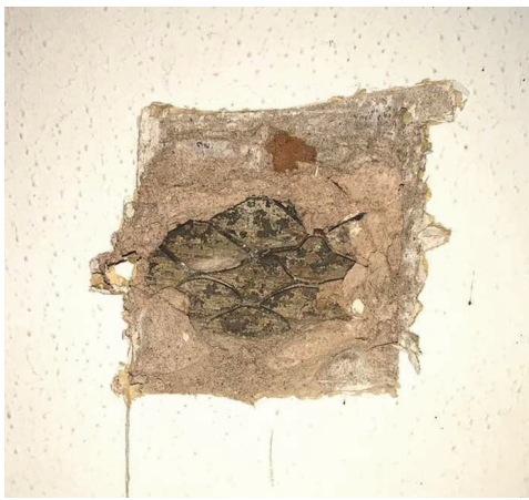
Figure 11 Wall makeup nearer boundary wall between living room and dining room.
