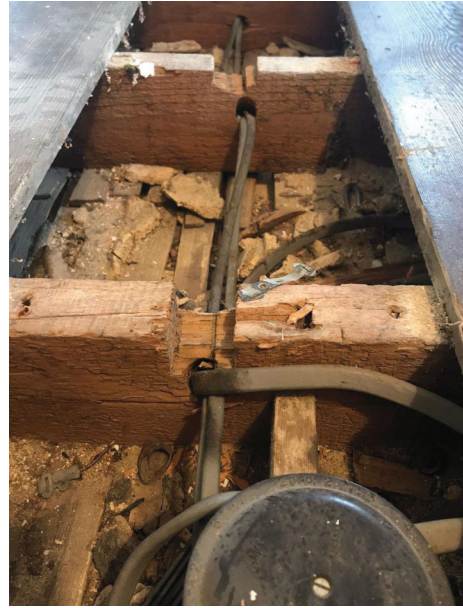
Figure 16 Existing First floor joists 2
