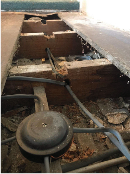
Figure 15 Existing First floor joists 1
