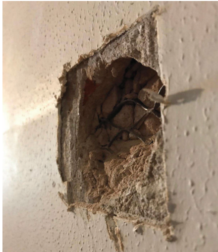
Figure 13 Wall between living room & dining room
