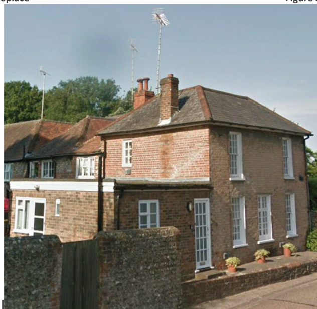
Figure 23 Chimney Brest from outside
