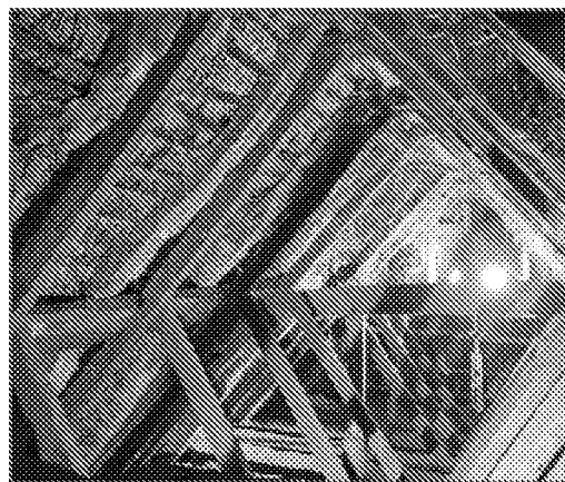
Roof structure with 1970s supportive structure.
