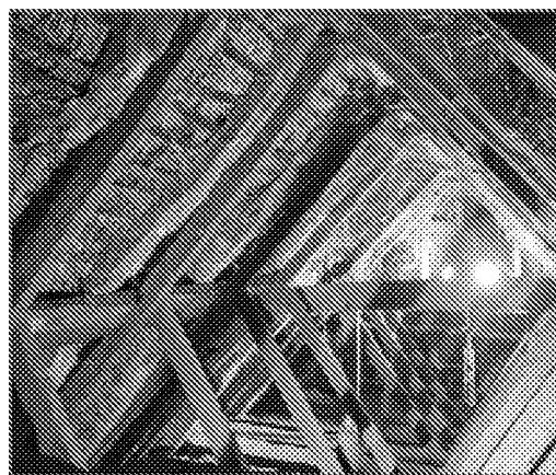
Roof structure with 1970s supportive structure.
