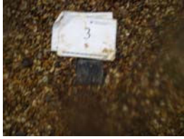
37. BH3 Made Good & installed
