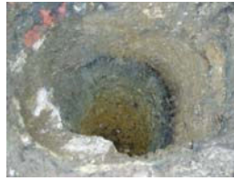
3. Starter pit BH1
