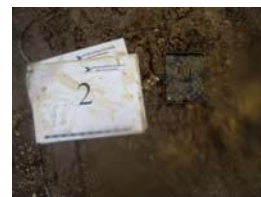
24. BH2 Made Good & installed
