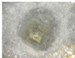
28. BH3 starter pit
