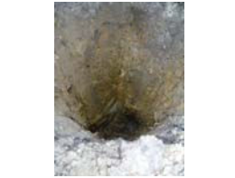
16. BH2 Starter pit
