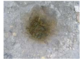
15. BH2 Starter pit
