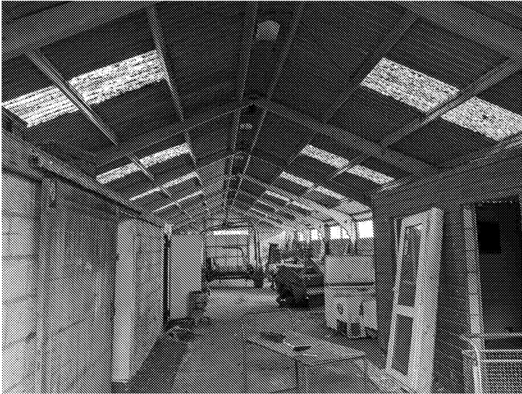
Photograph 5 - Inside of B03. Heavy use by birds on fat roofs to right and left.
