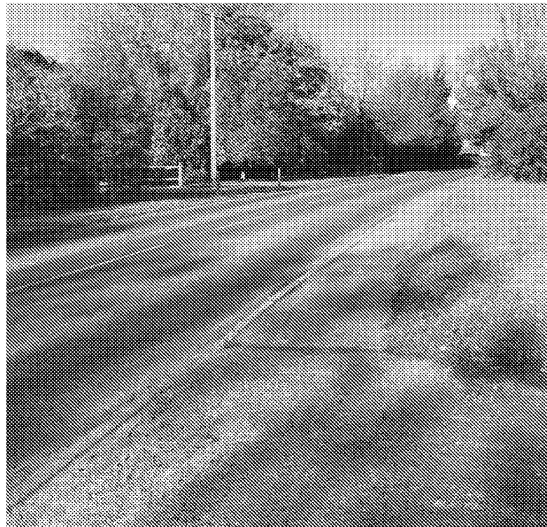
Photograph 3. Visibility to the north at a 2.4m set back from Yaptan Road Carriageway
