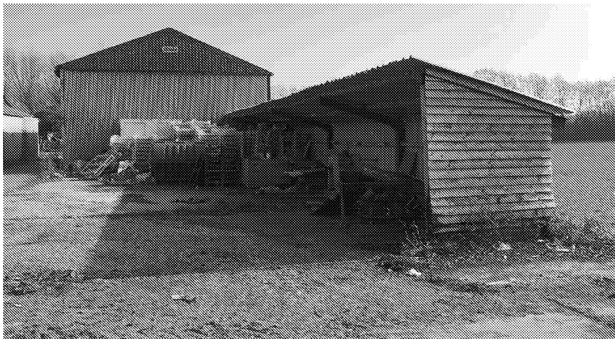
Photograph looking south-east towards the existing open-fronted building.
