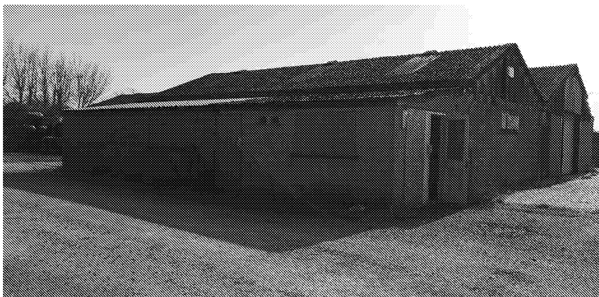
Photograph looking south-east showing the existing agricultural buildings.
