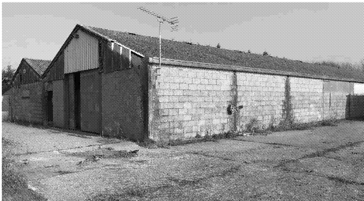
Photograph looking north-east towards the existing agricultural buildings.
