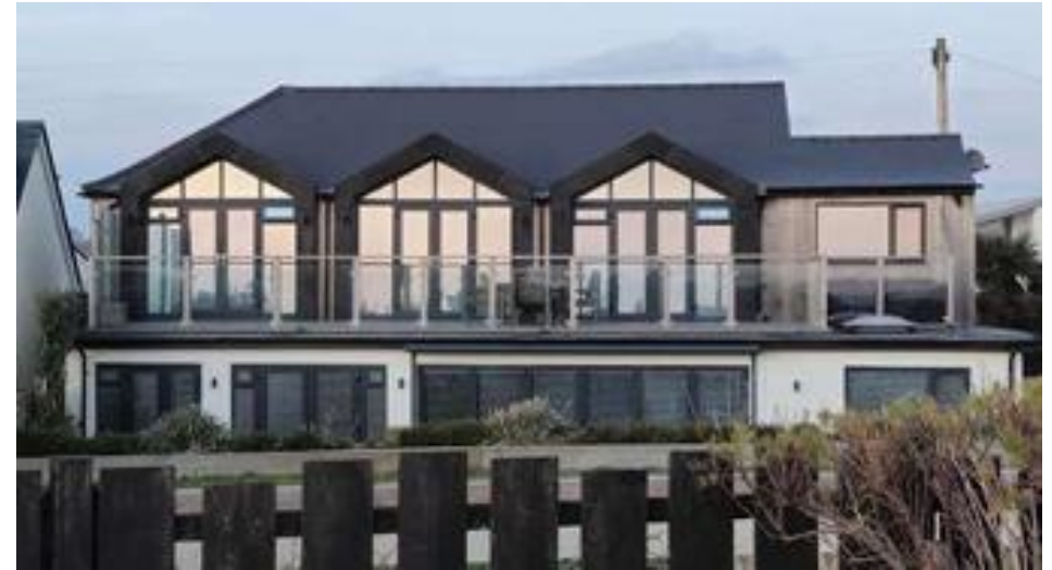
Dwelling with glazed and metal railed balcony at first floor Level and sat upon a flat roof structure
