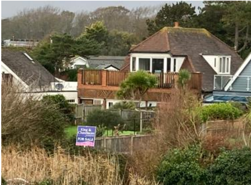
Dwelling with fully timber balcony – open sided beneath, located to the west of the application property
