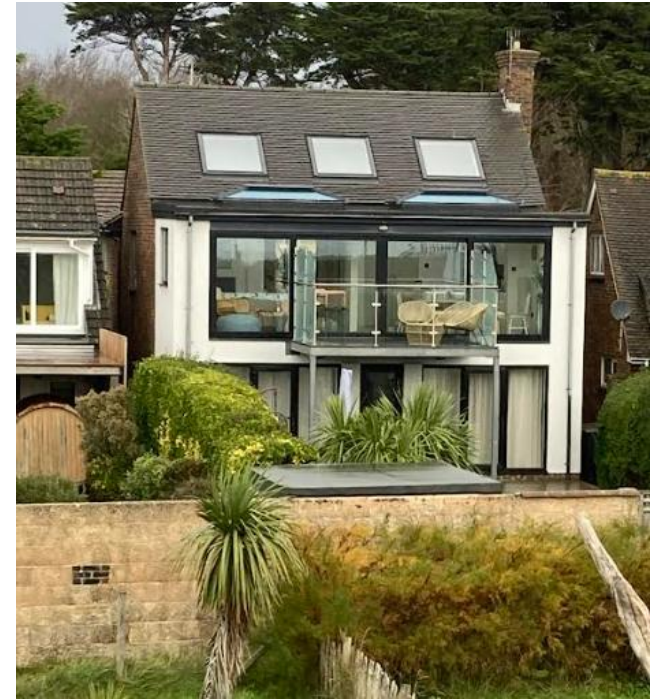
No. 2 Elmer Court, to the east of the application property
