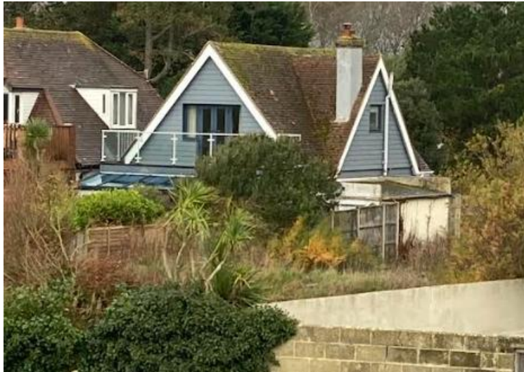
Dwelling with glazed and metal railed balcony, set upon a single-storey, lean-to structure, located to the west of the application property
