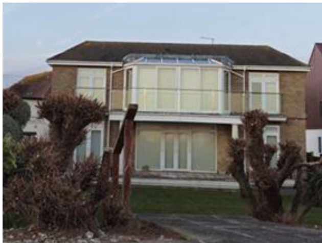
Dwelling with metal railing and balcony sat upon a masonry structure – open sided beneath, located to the west of the application property
