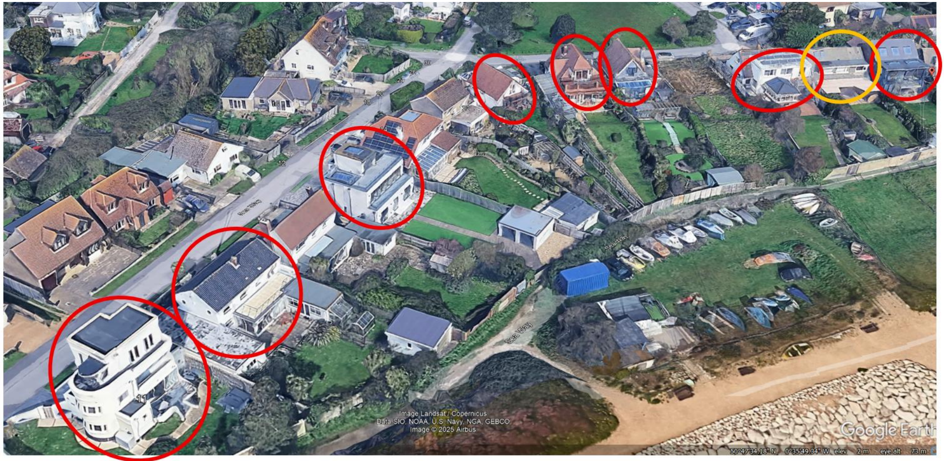
The above aerial imagery identifies, in red, dwellings with balconies within the immediate vicinity of the application dwelling (highlighted in yellow) - Source: Google Earth Pro
