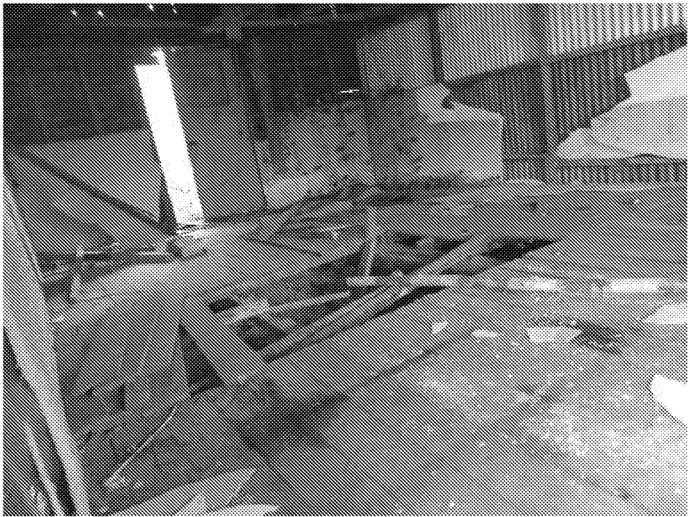
Photo 15: Typical large shed interior
