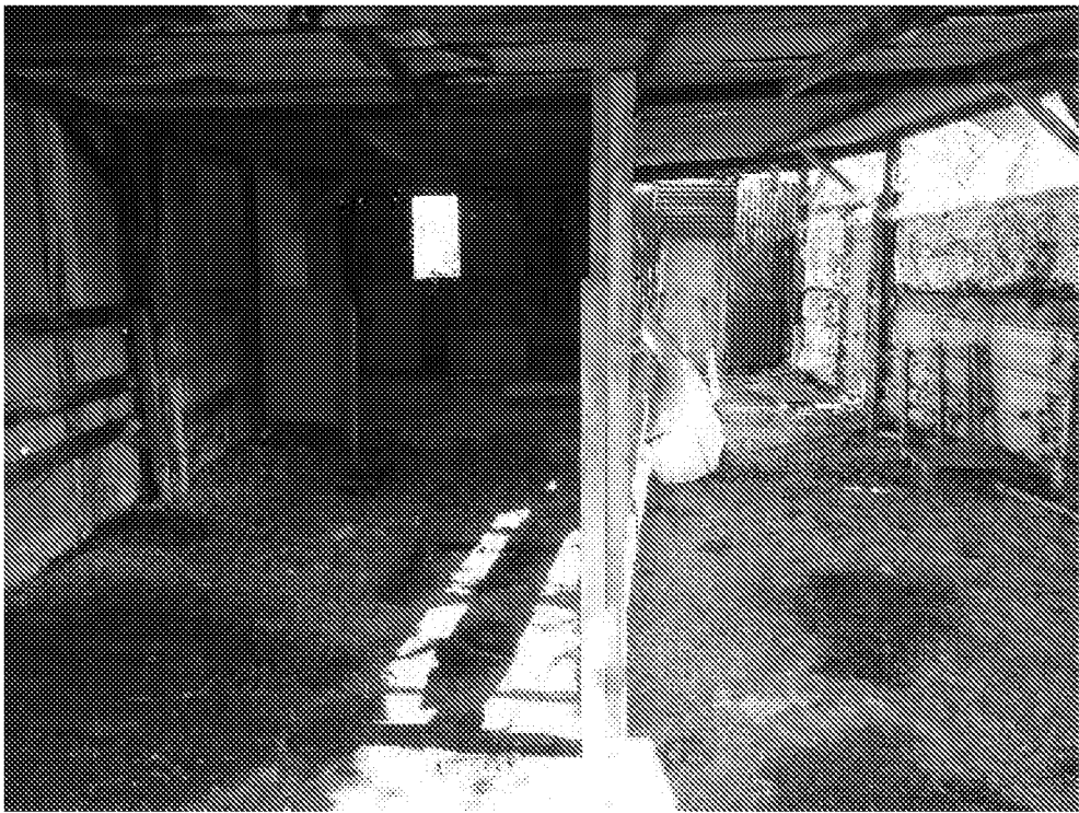
Photo 14: Typical large shed interior
