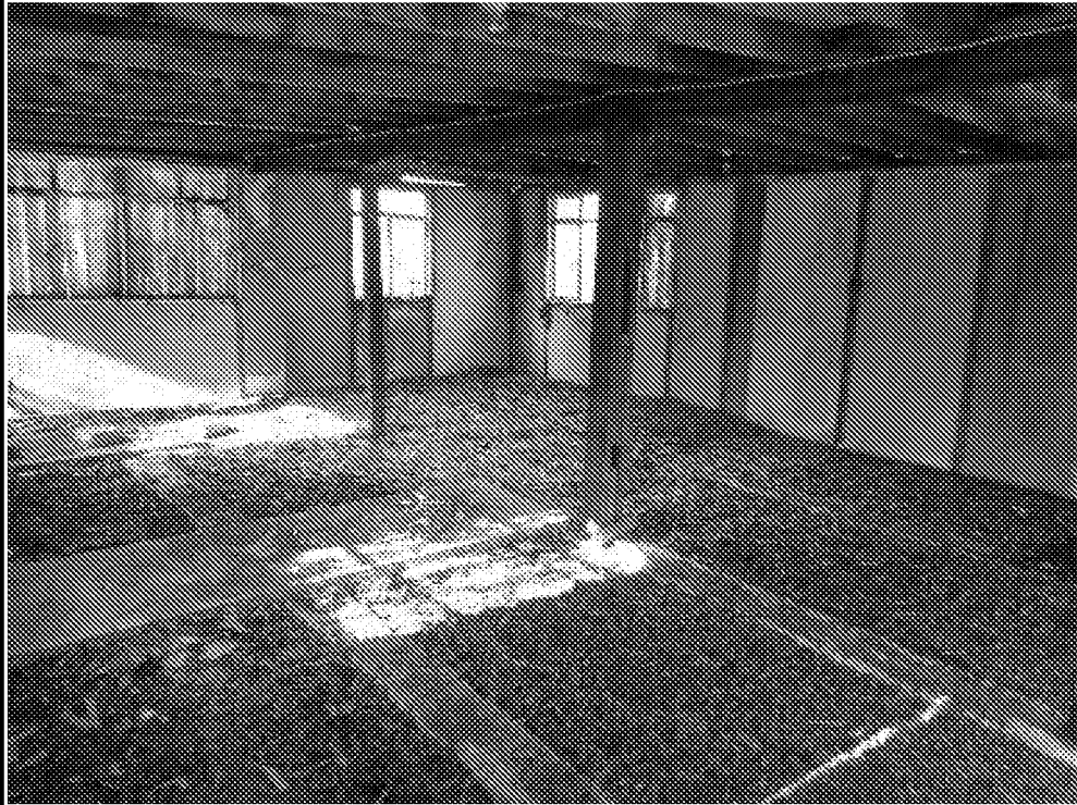
Photo 16: Typical large shed interior
