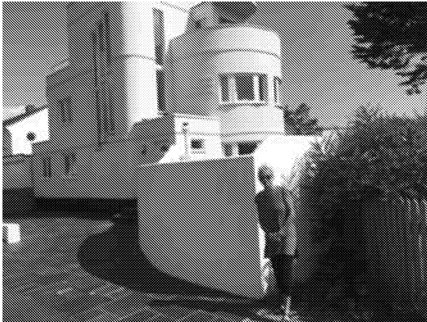
Photograph 05 showing a similar boundary wall in the vicinity
