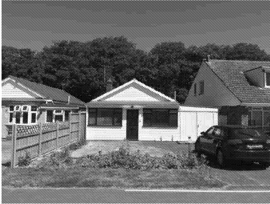
Photograph 01 showing the existing front elevation
