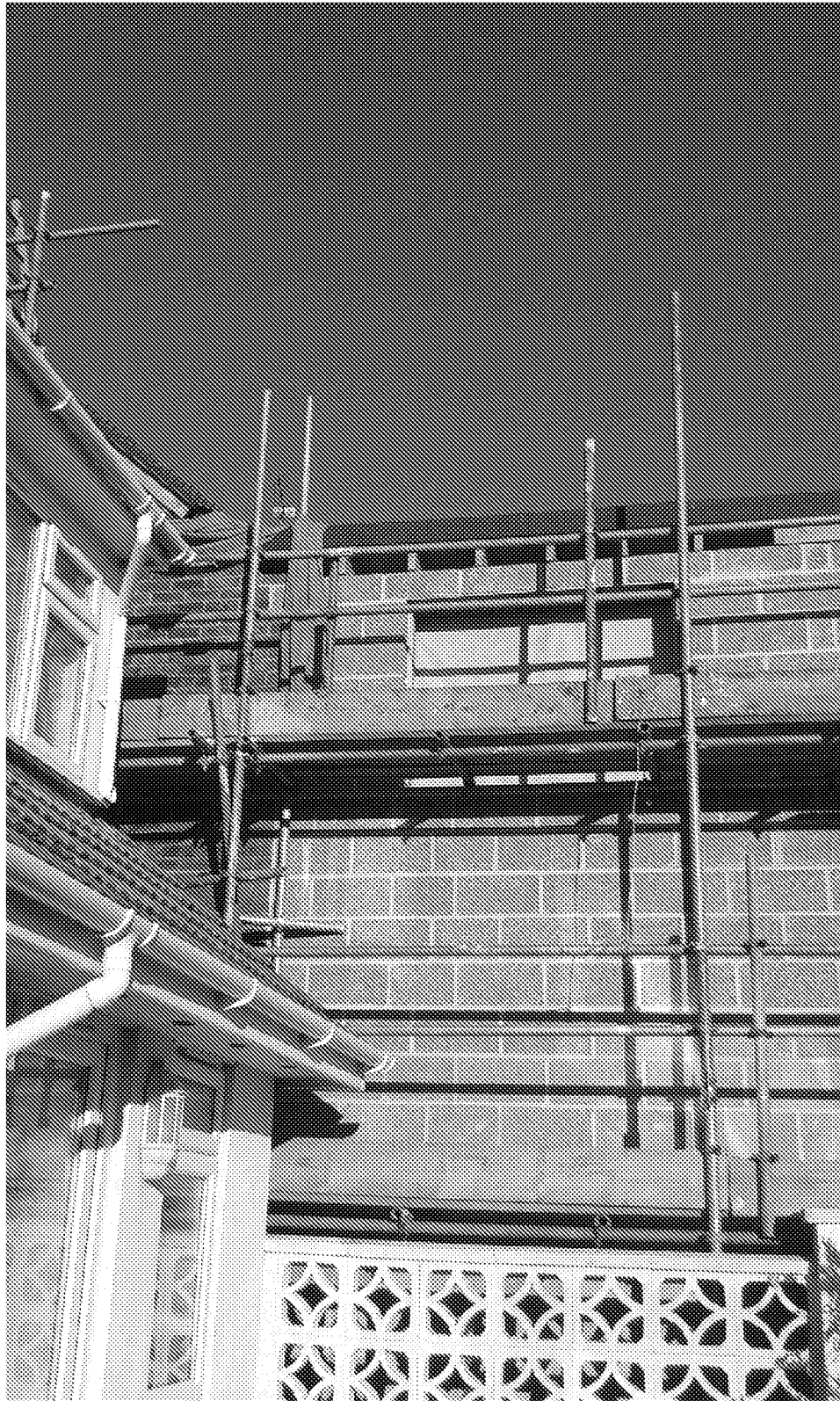
The photograph above shows the relationship of the side window with the rear facing window of his youngest child's bedroom, during construction.
