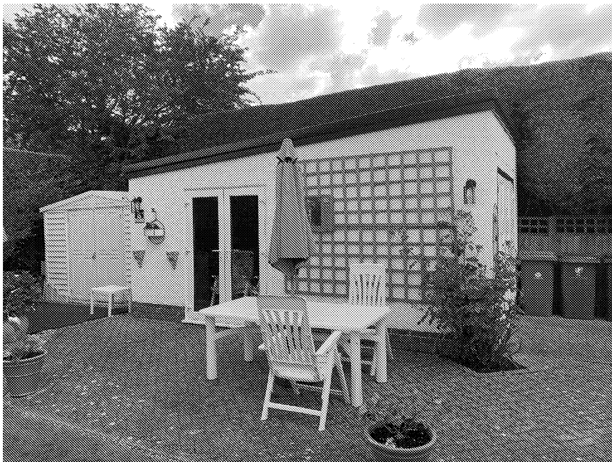
Pic – View of the current garage with the Hawthorn and Leylandii hedges.
