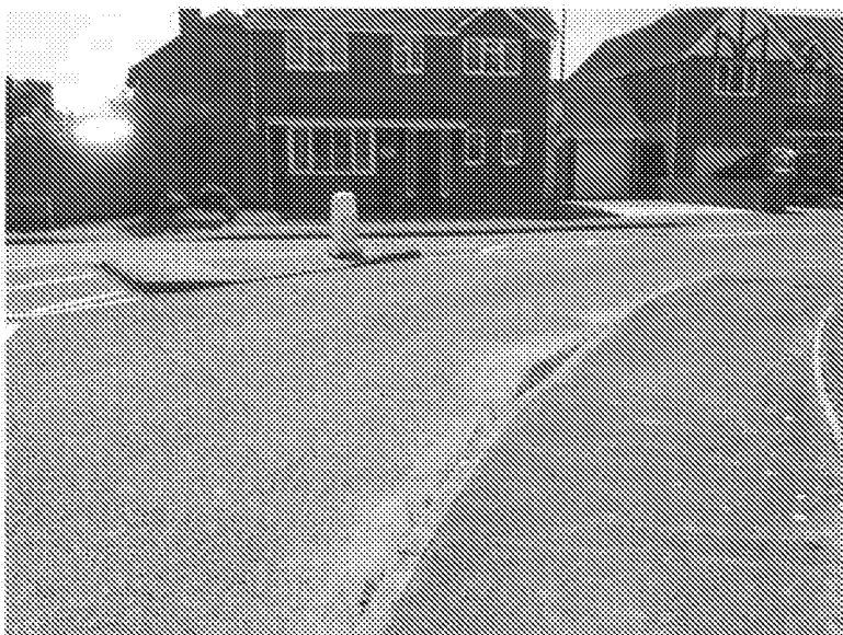
Figure 4-4 Silver Birch Drive -- View South-West
