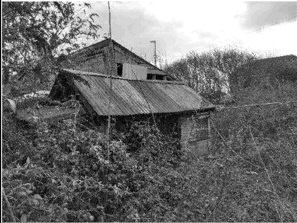
Photo 13: Typical large shed construction
