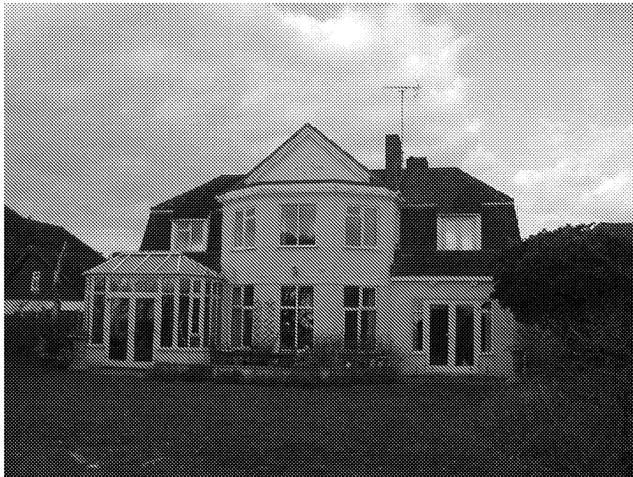
Pic. – View of the rear of the existing dwelling.
