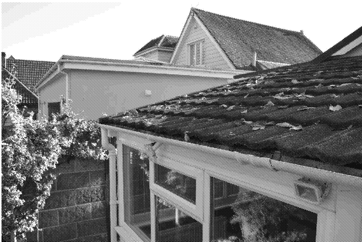
Rear view showing large rear extension to no.90 Ancton Way beyond
