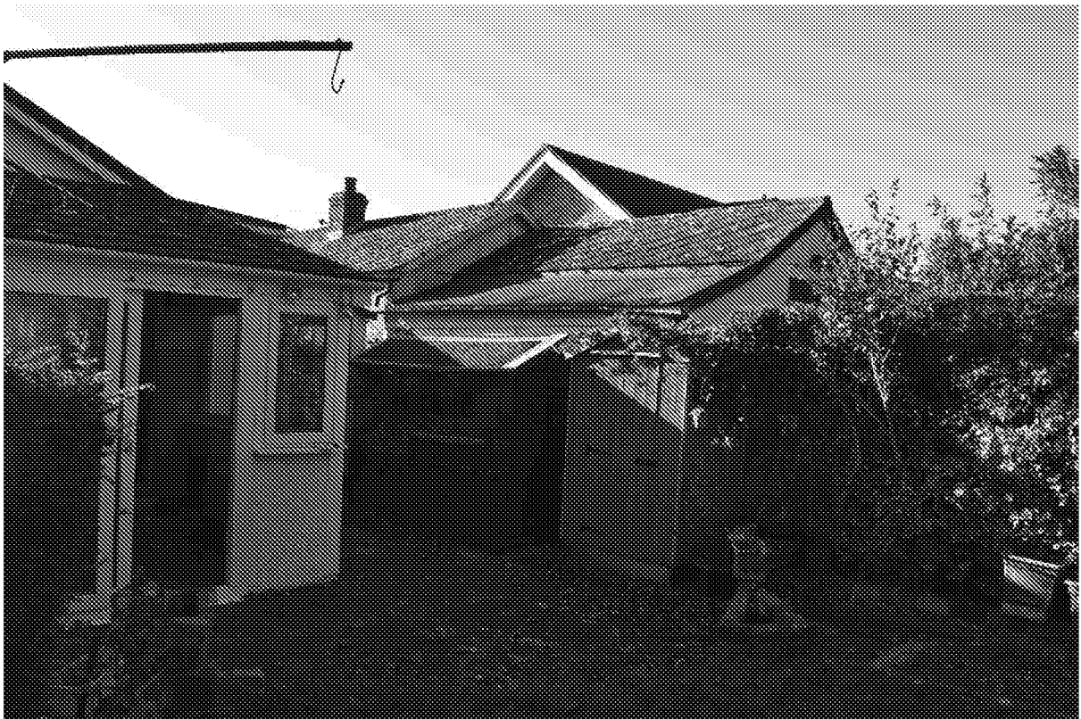
Rear view showing extensive roof scape to neighbouring bungalow no.86 Ancton Way beyond
