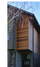
B - WEATHERBOARD CLADDING
