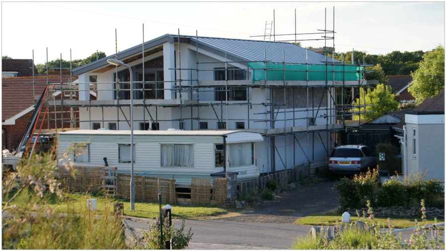
6 ALLEYNE WAY - ZINC ROOF MODERN STYLE REPLACEMENT DWELLINGS - ELMER SANDS ESTATE
