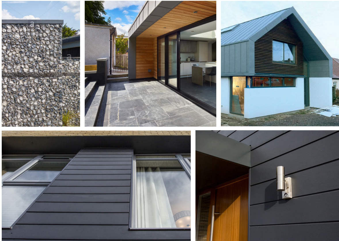
Fig 4. examples of flint, zinc cladding, render and fibre cement cladding
