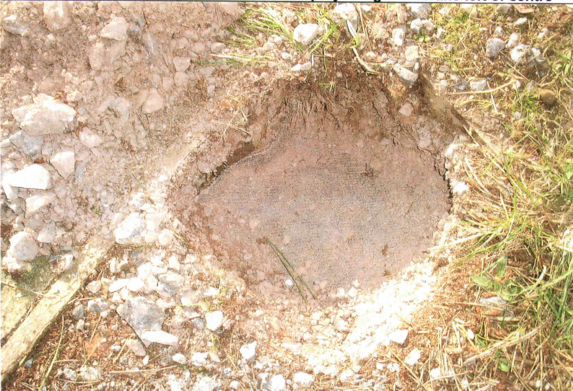
B. Excavation to establish base
