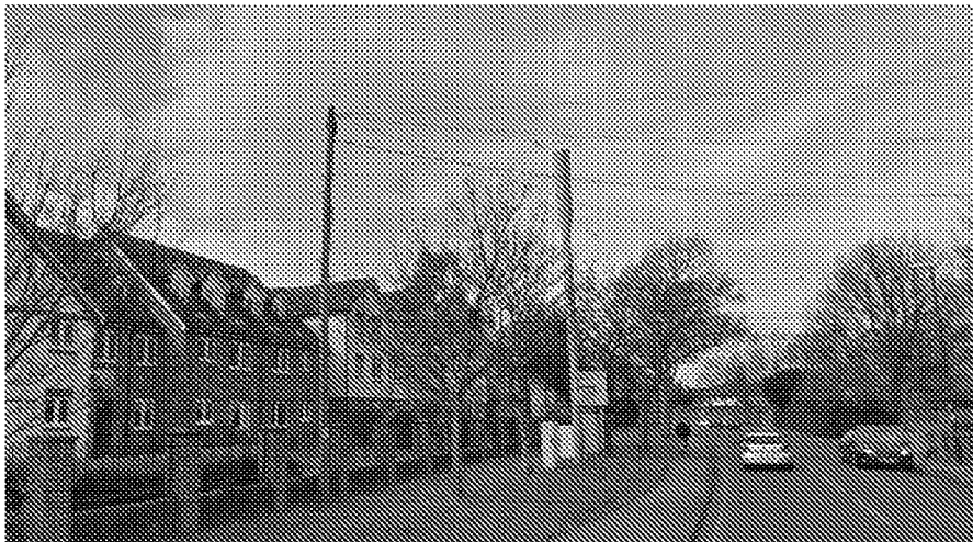
Image 1: Existing 2G/3G/4G site
