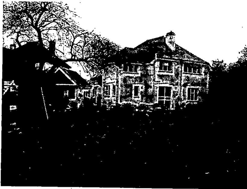
Rear of building to be extended.
