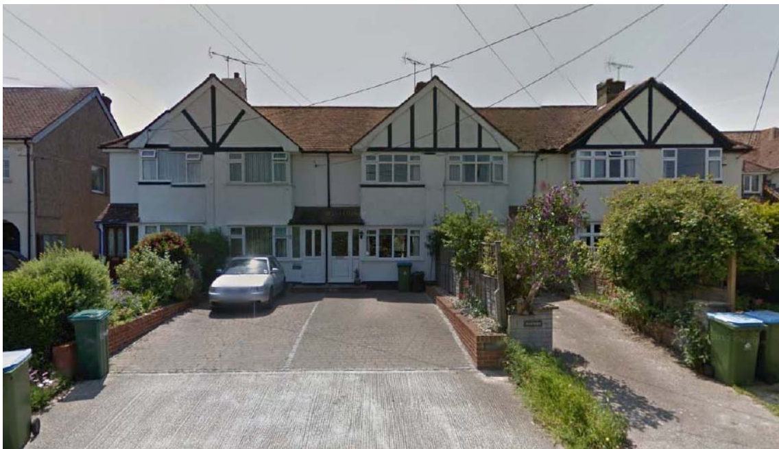
Figure showing common white render finish on Ancton Lane.
