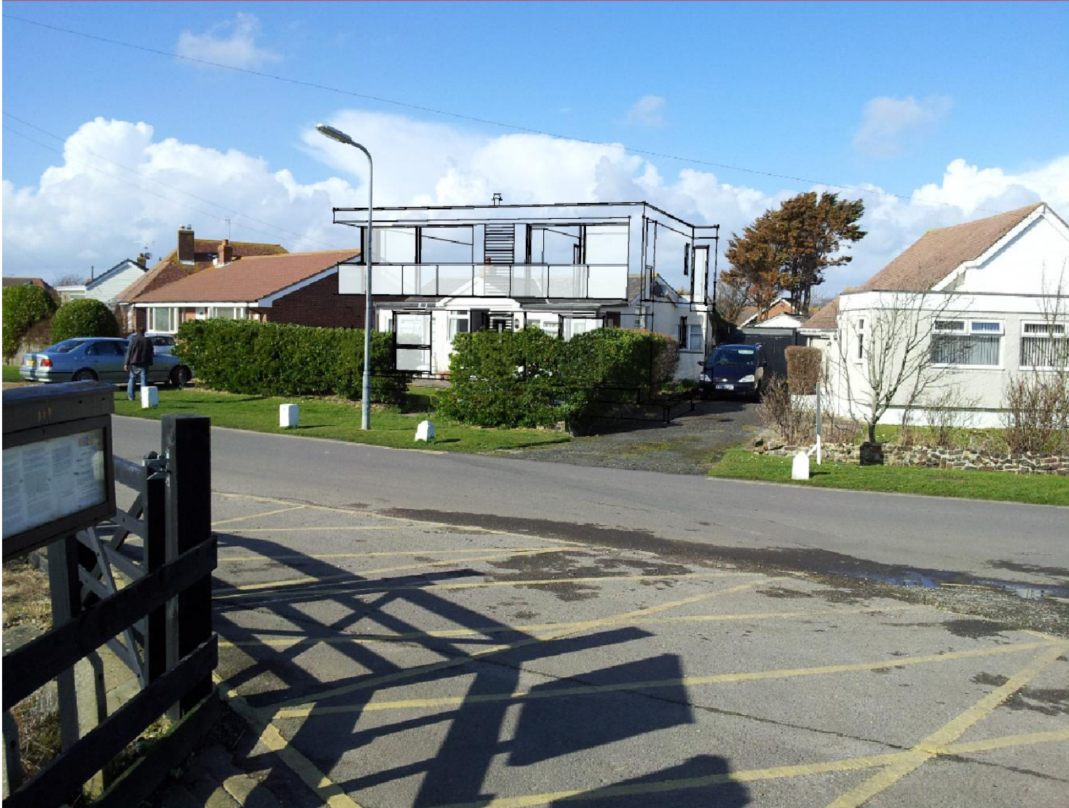
Replacement House 6 Alleyne Way Elmer Sands Middleton PO22 6JZ Street Scene #2
