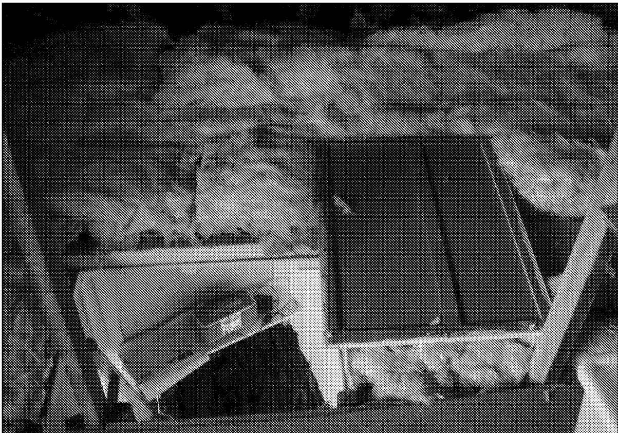
Photograph 7. Showing glass-fibre insulation and hatchway within the attic of the bungalow.
