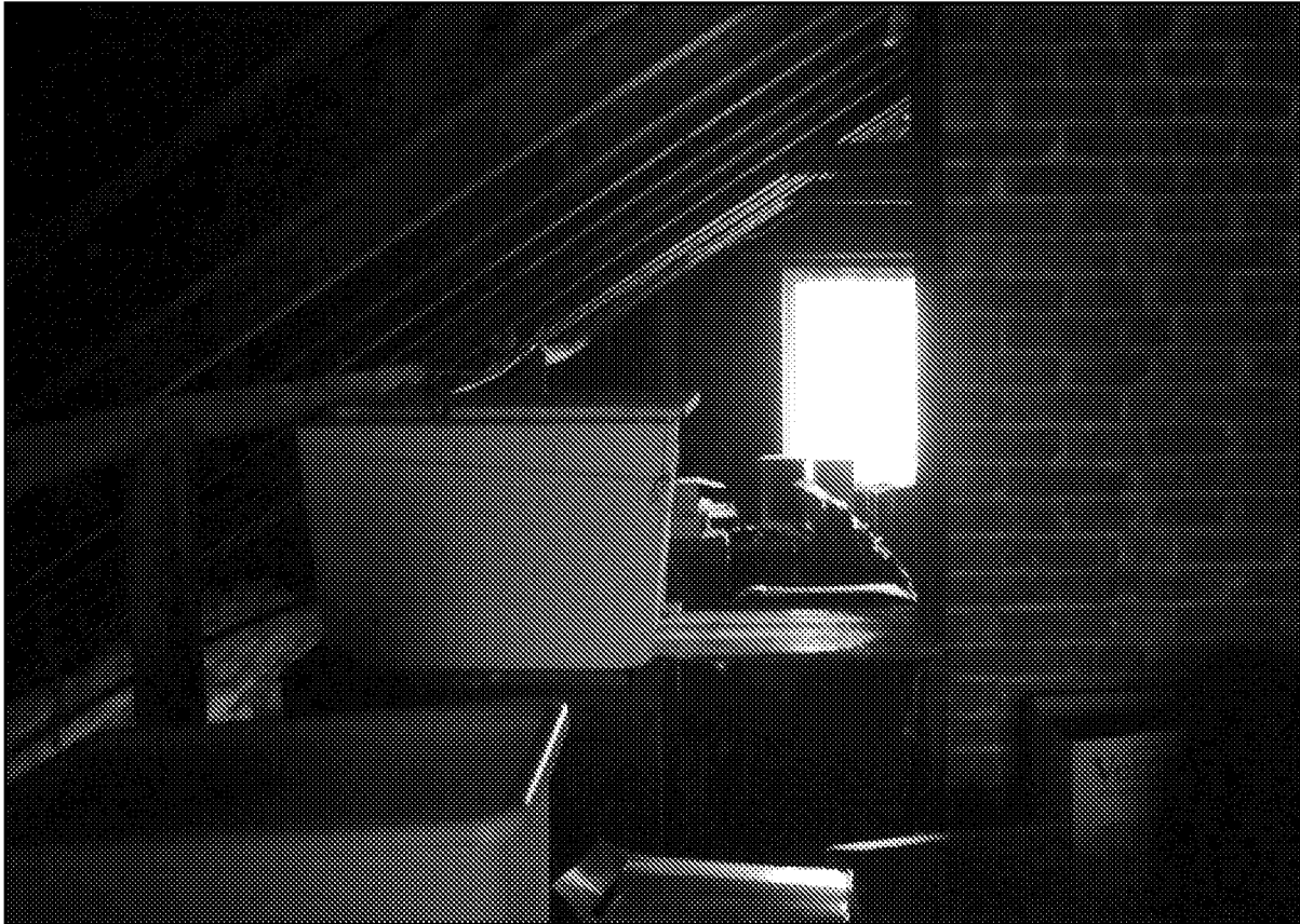
Photograph 6. Showing a water tank beside the chimney stack within the attic of the bungalow.
