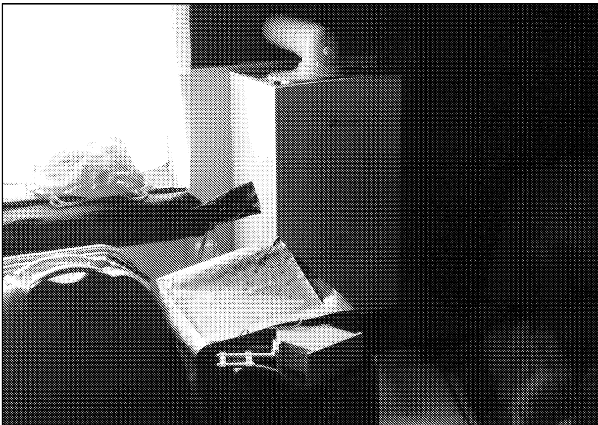
Photograph 9. Showing the gas boiler on the northern gable, within the attic of the bungalow.
