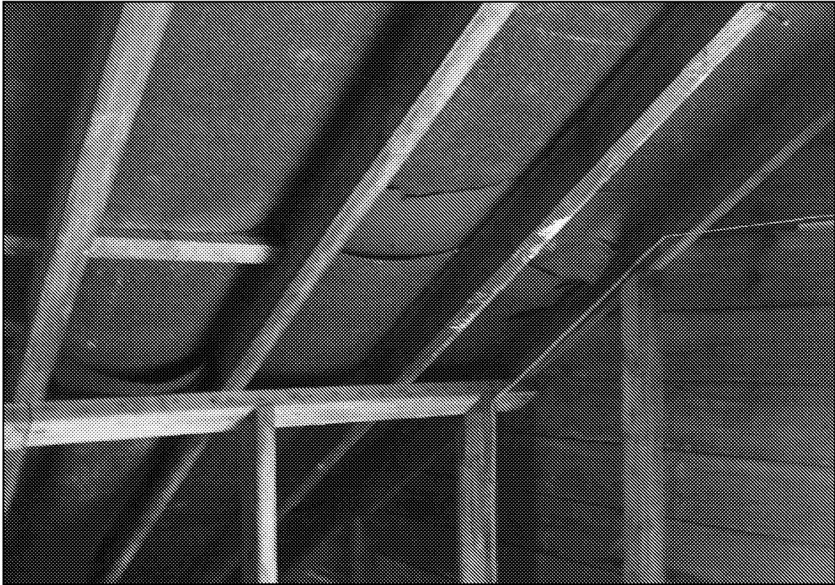
Photograph 8. Showing bitumen felt lining and timber gable cladding, within the attic of the bungalow.
