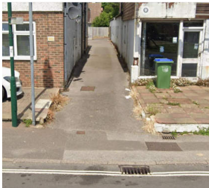
Figure 7. Existing gullies in the footway and carriageway, collecting run-off from the existing access drive
