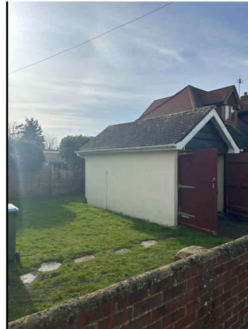
existing garage building
