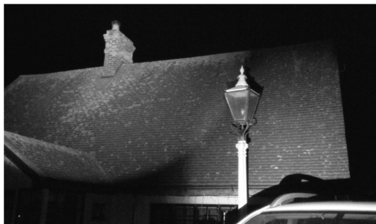
B1: A view of the eastern elevation.
