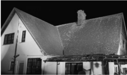
B1: A view of the western elevations.
