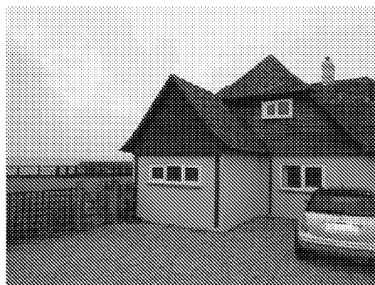
Extension on eastern end of house
