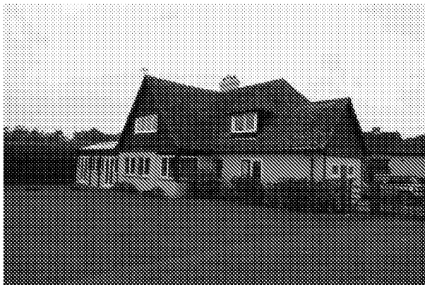
Southern aspect and eastern side
