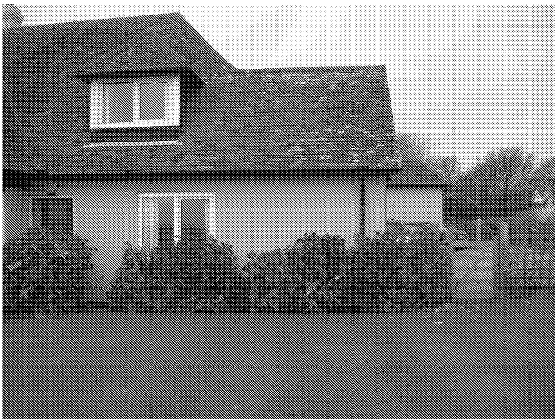
Photo 3: Lawn and side-wing of property to be demolished
