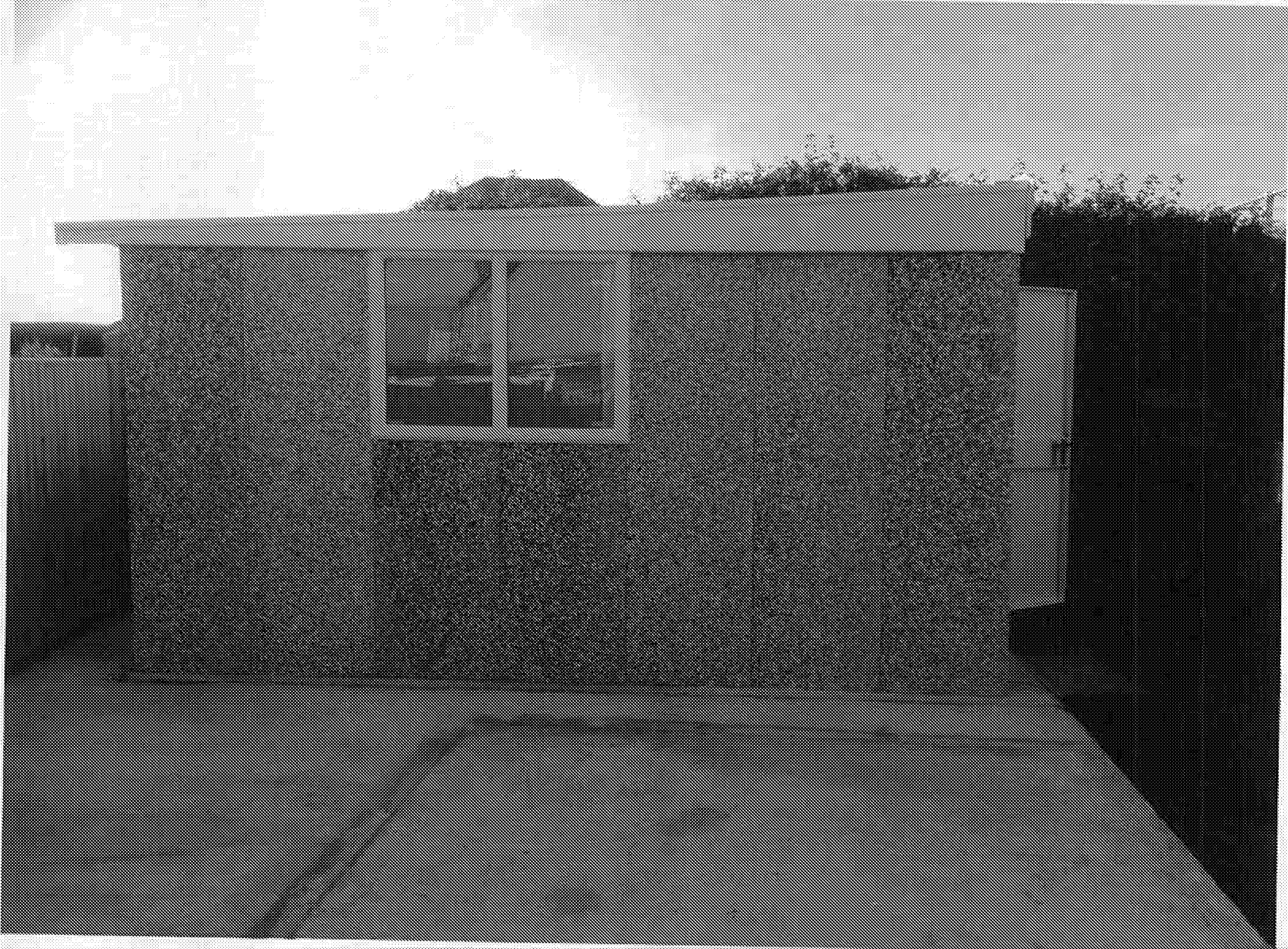
Taken when our shed was completed autumn 2017.
