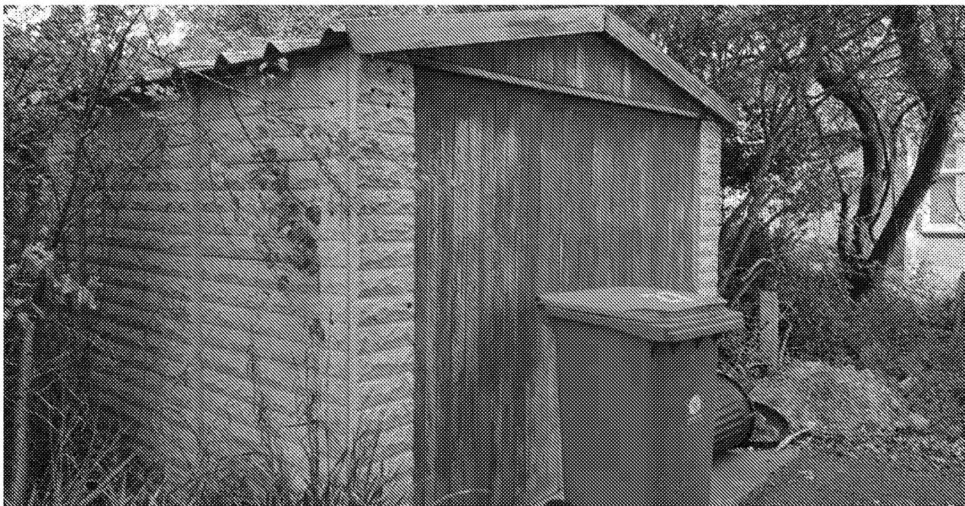
Photograph No. 05 - Building B2; assessed as offering negligible bat roost suitability.
