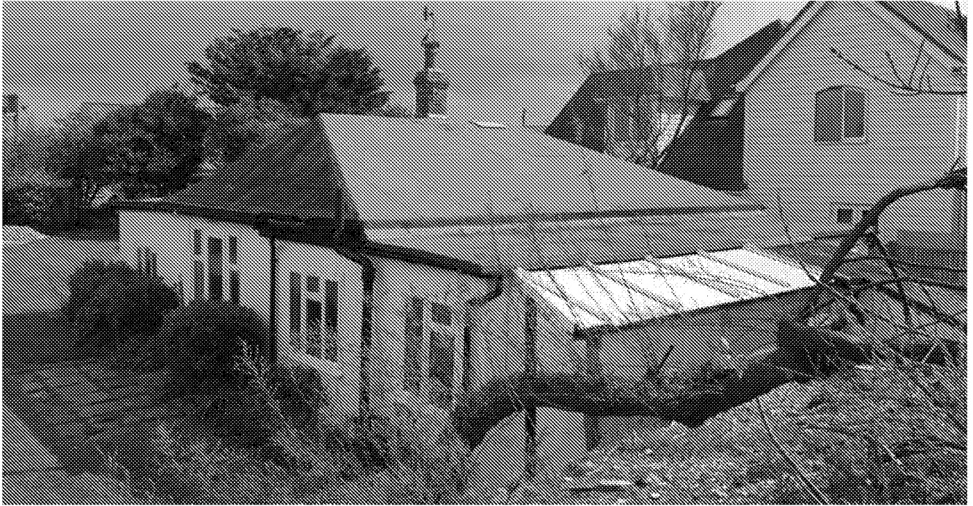
Photograph No. 03 - Building B1, assessed as offering negligible bat roost suitability.
