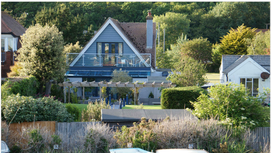
2 THE HARD REAR ELEVATIONS OF PROPERTIES - THE HARD & ELMER COURT
