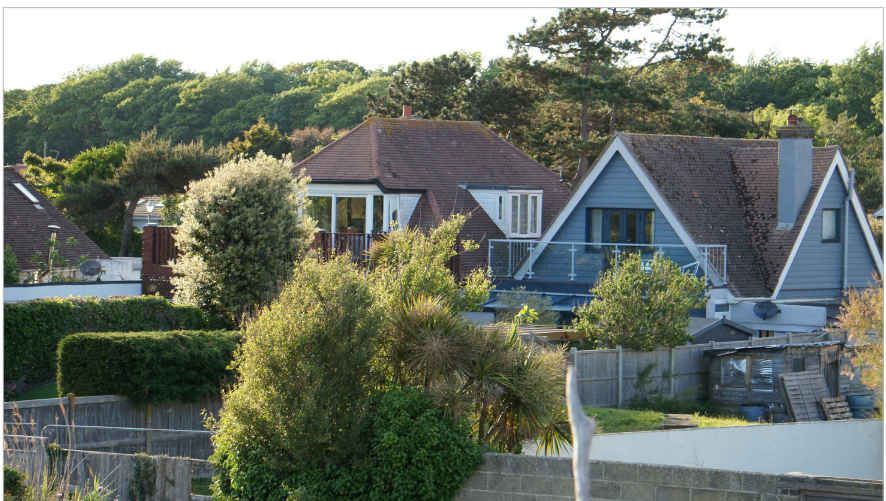
1 & 2 THE HARD REAR ELEVATIONS OF PROPERTIES - THE HARD & ELMER COURT
