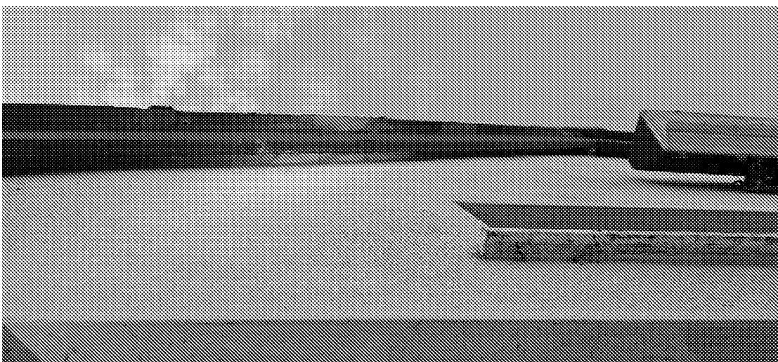
Photo 9 – Northern gable end showing roof tiles oversailing with well-sealed timber
