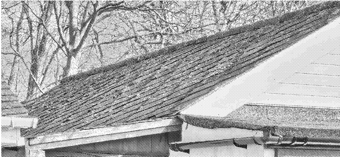
Photo 7 – West roof pitch with flat fibreboard tiles
