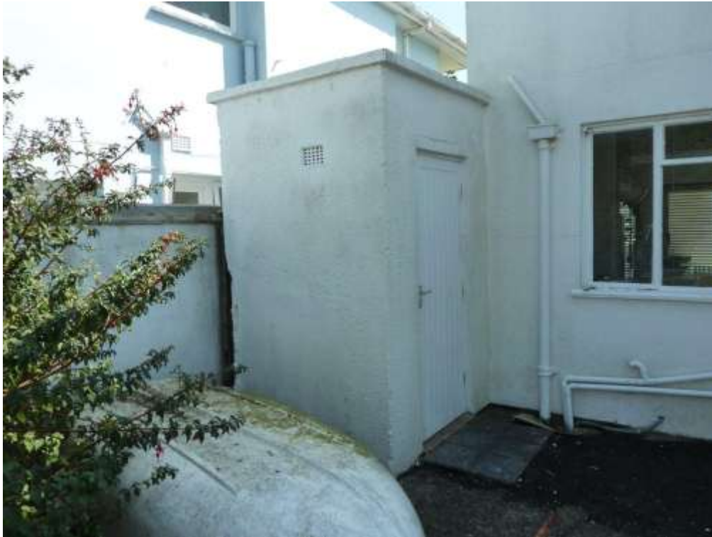
North East corner – Single storey extension to be removed
