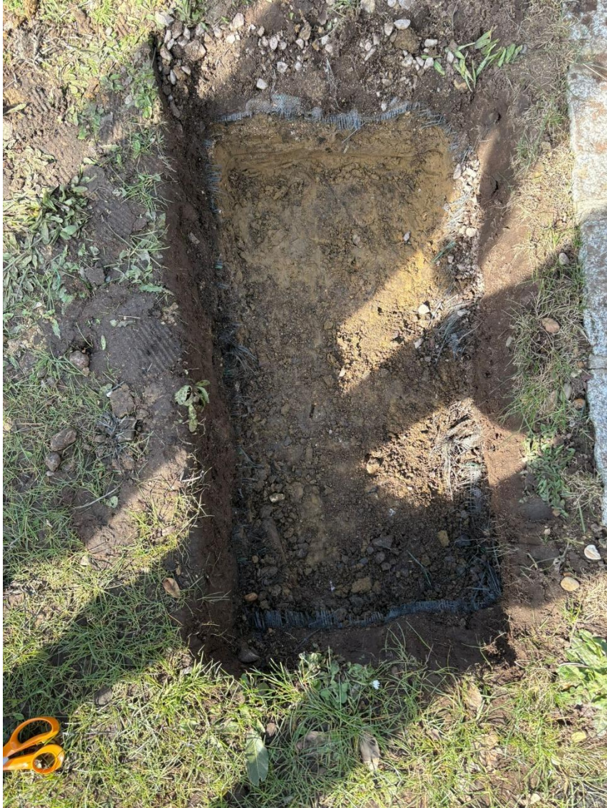
Soakage pit excavated at front (driveway)
