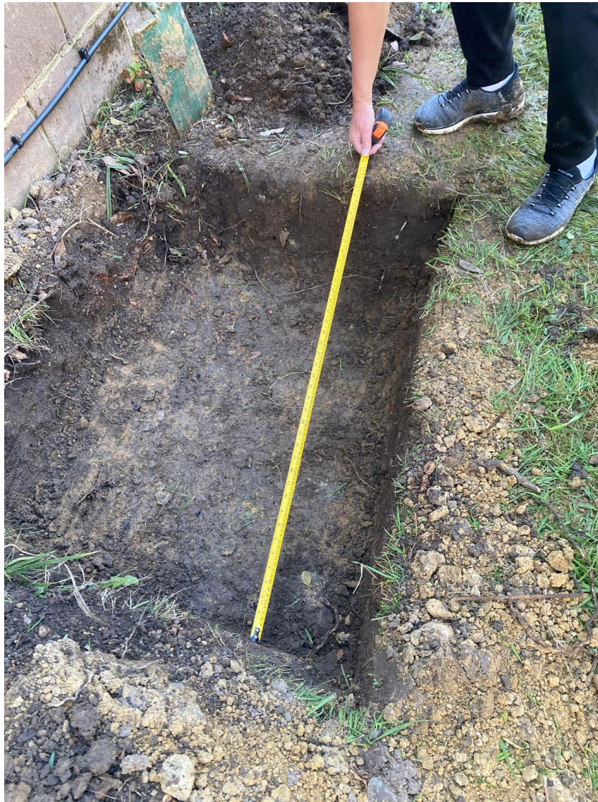
Soakage pit excavated at rear (rain gardens)
