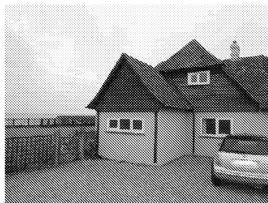
Extension on eastern end of house
