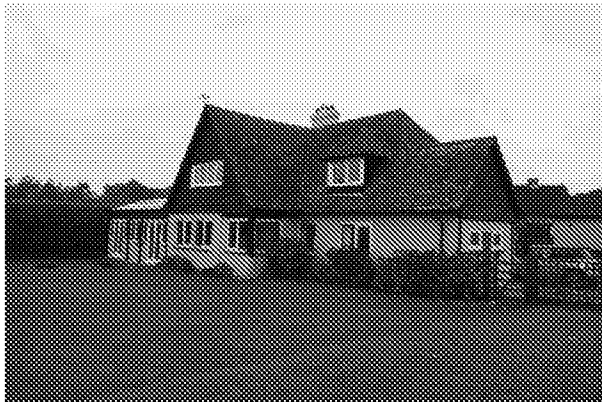
Southern aspect and eastern side
