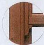
Run through sash horns
