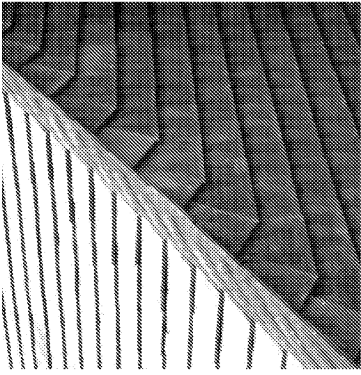
Plain clay tiled dormer roof with bonnet hip tiles and tile hung dormer cheeks
