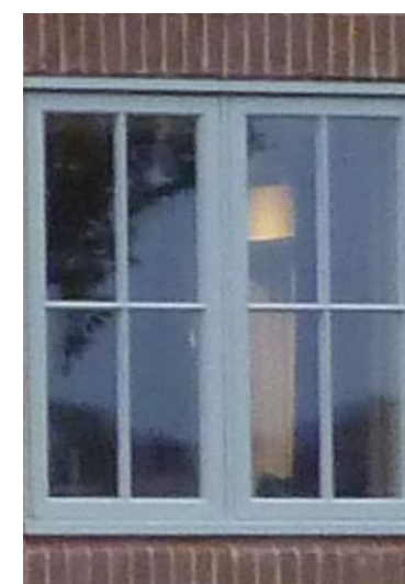
Grey window frames with head and cill feature brick courses
