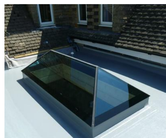
Lead Grey coloured GRP flat roof membrane with roof lantern
