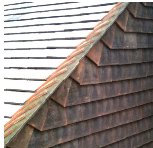
Example of plain clay tile hanging with Winchester cutting at verge
