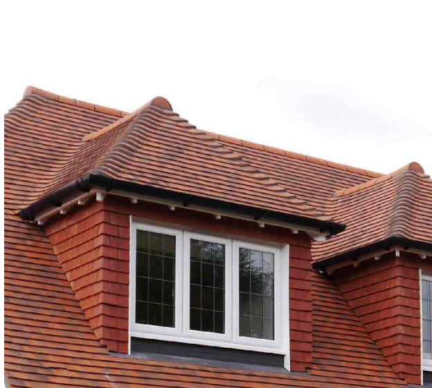
Plain clay tiled dormer roof with bonnet hip tiles and tile hung dormer cheeks
