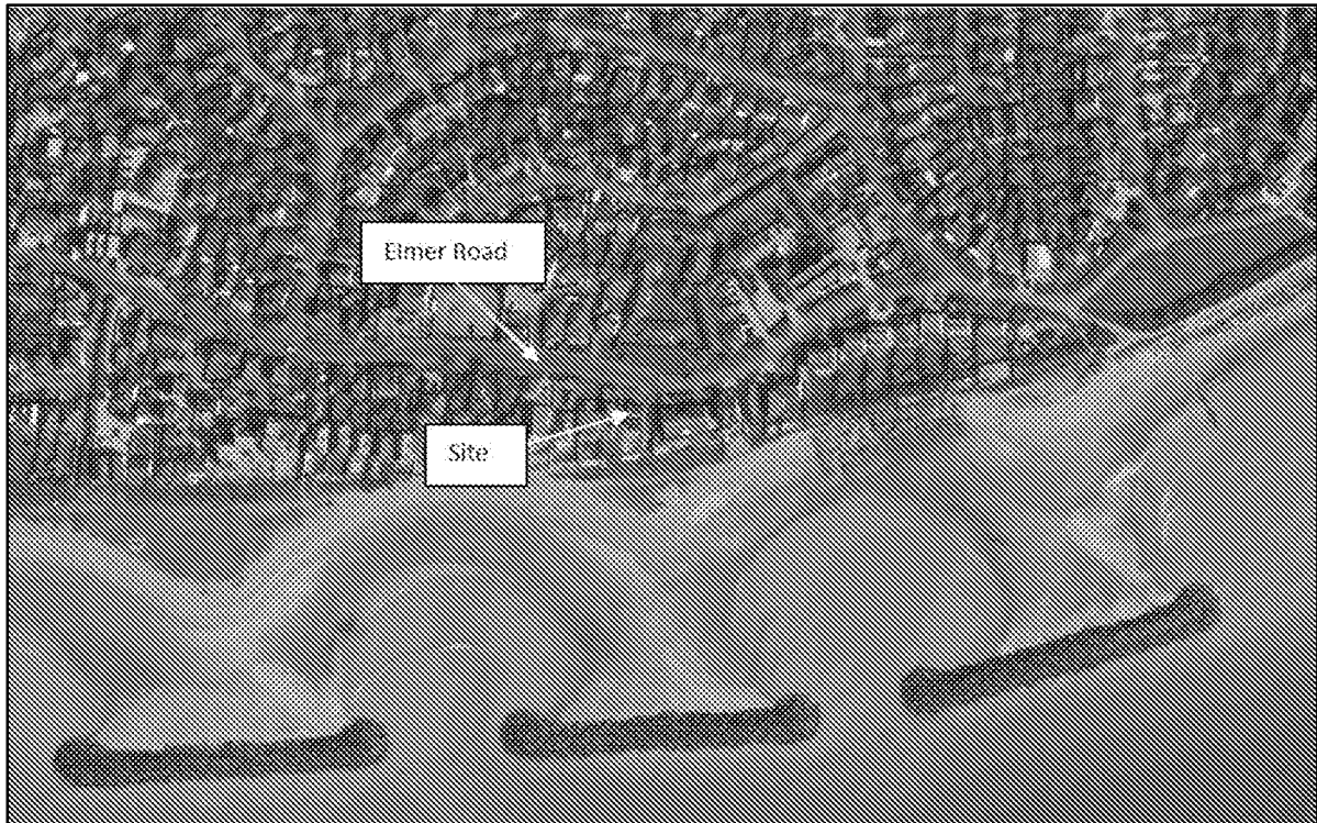
Figure 2: Aerial imagery, showing location of site (Source: Google Satellite)
