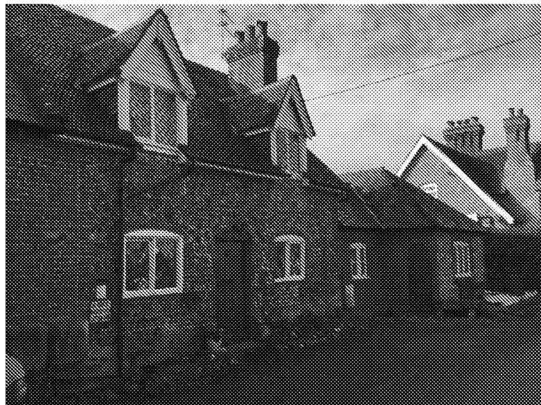
Front elevation from Church Lane (looking East)
