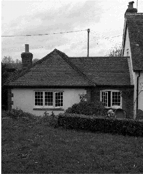
Rear Elevation: Single storey wing.
