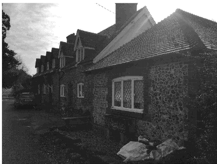
Front elevation from Church Lane (looking West)
