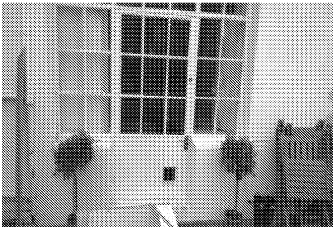
Present Door to Conservatory from House – 1928 original door opening (to be fully retained)
