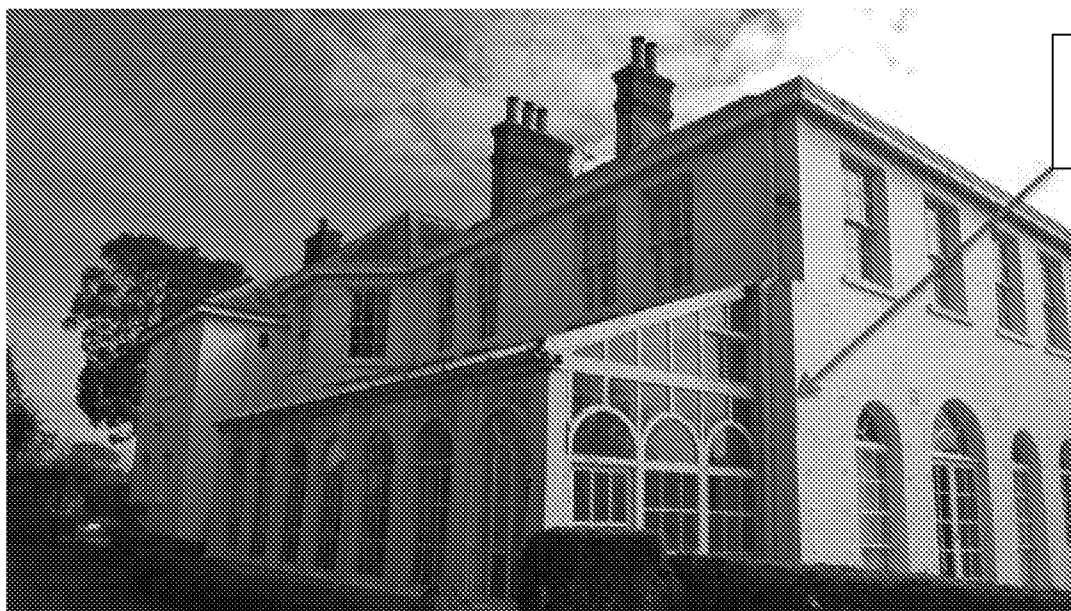
Photo of south westerly conservatory junction elevation of Lyminster House
