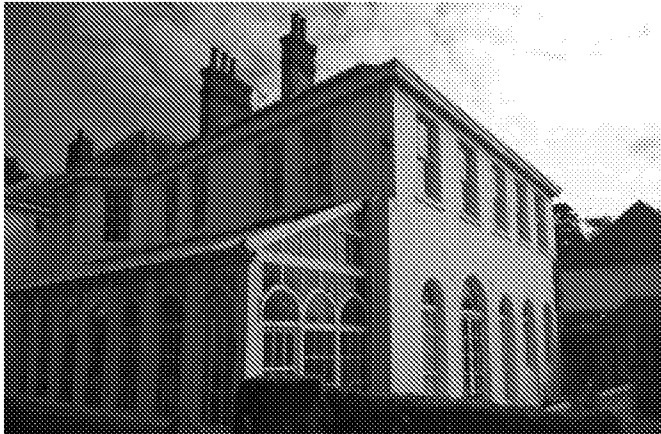
External Conservatory façades – Southwest – 1928 extension which also incorporated the construction of the present conservatory structure
