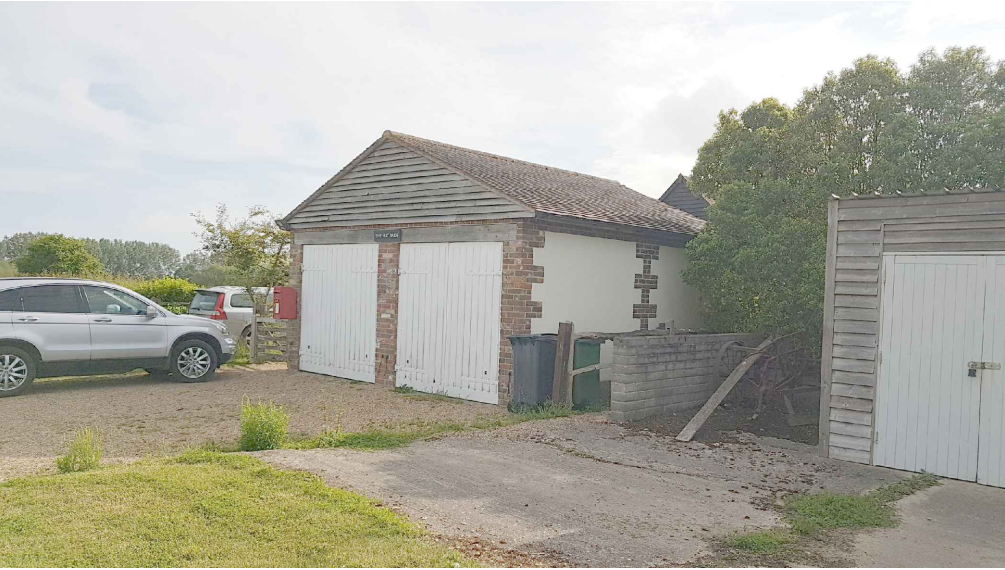
4> Looking West: view of front of neighbouring out buildings and boundary.
