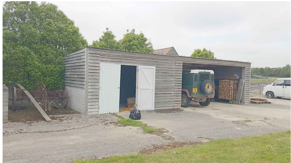
5> Looking North-West: view of front of out building and fence behind.
