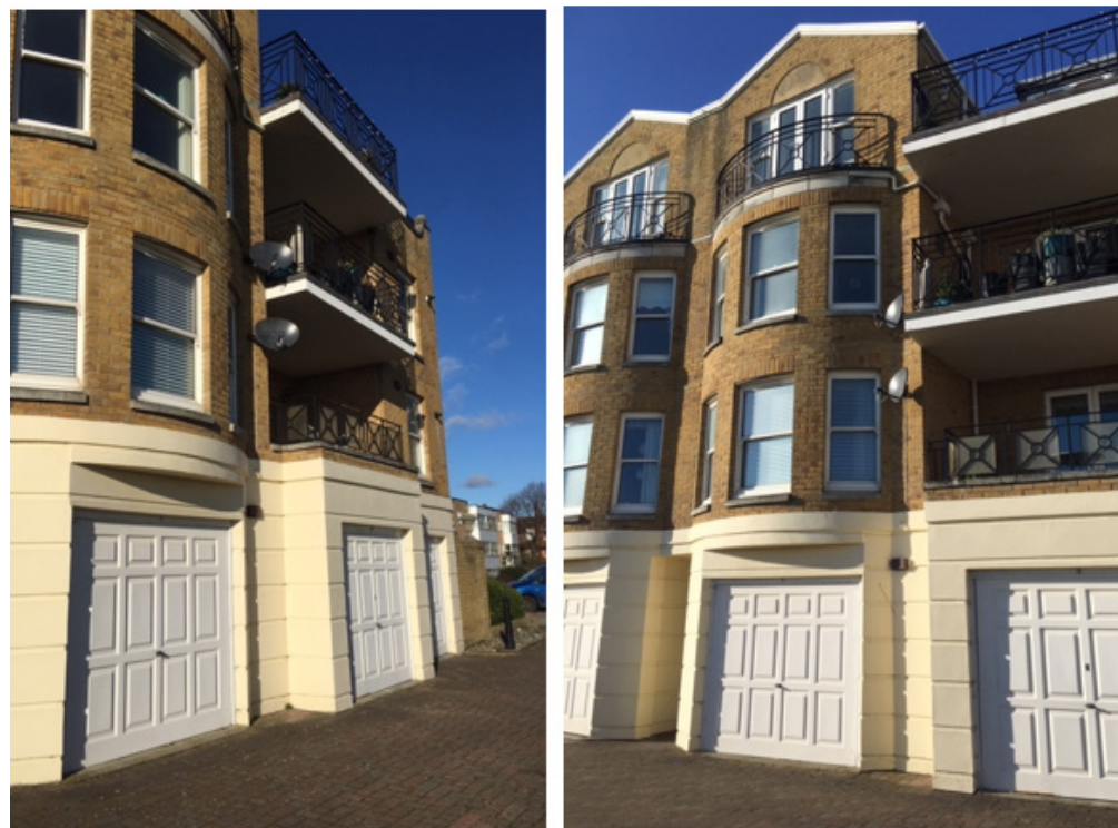
Extent of flats seen from service road demonstrating the existing French doors set back from the balcony edge and as such cannot be seen from the rear service road
