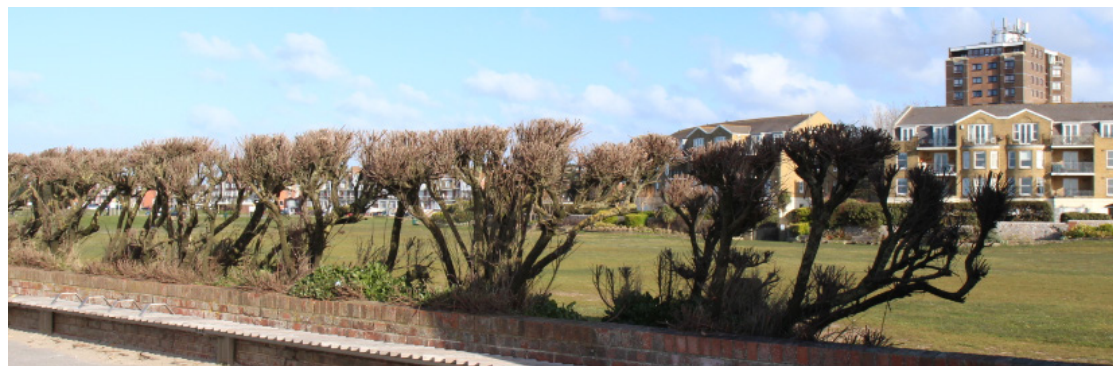
Beach Crescent block seen from the promenade
