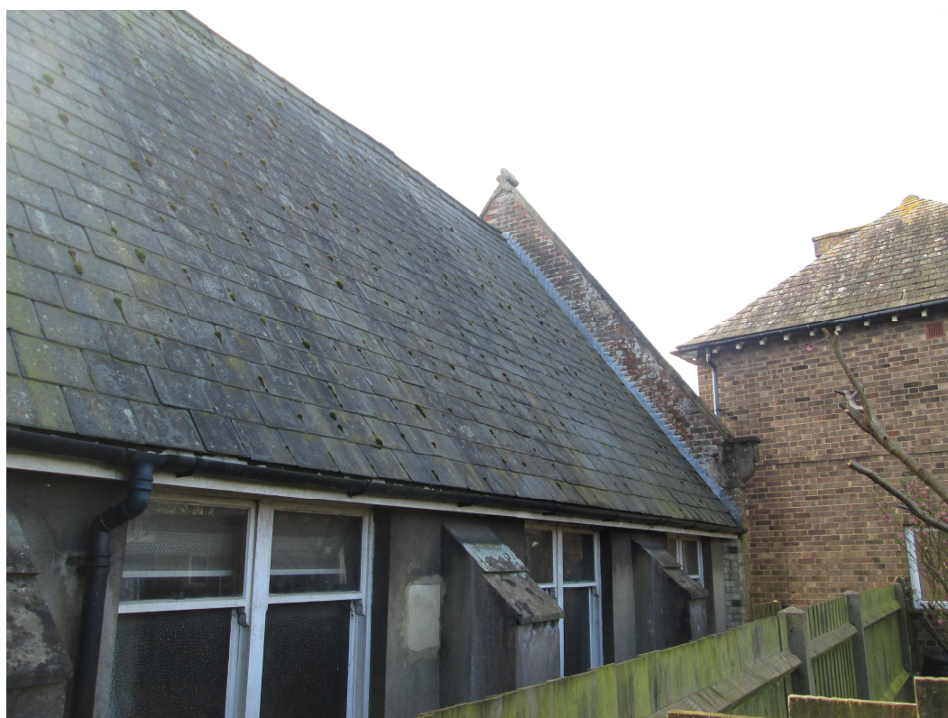
North Wall of Knight Hall as existing
