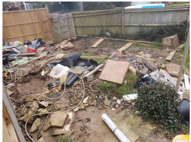
Soakaway located in middle of pic
