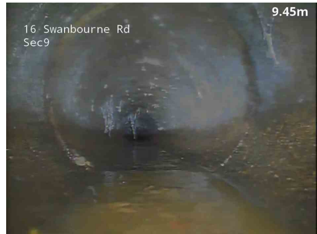
4, 00:00:21, 9.50 m Attached deposits, fouling from 4 o'clock to 8 o'clock, 10% cross-sectional area loss, finish
