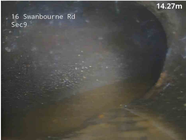
7, 00:01:09, 14.40 m Finish node, major connection without manhole, reference: Sewer
