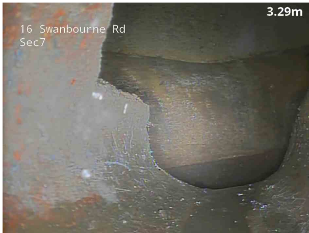
3, 00:00:24, 3.30 m Finish node, manhole, reference: MH1
