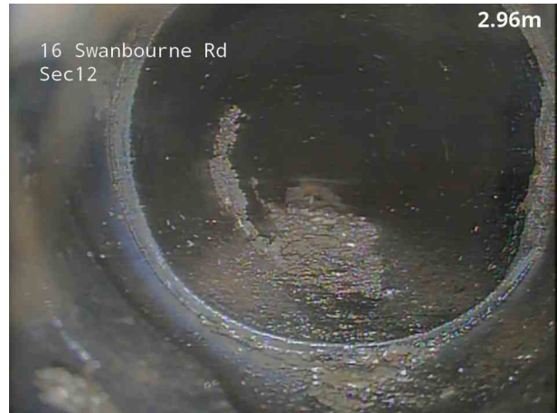
2, 00:00:33, 3.10 m Settled deposits, fine, 10% cross-sectional area loss, start
