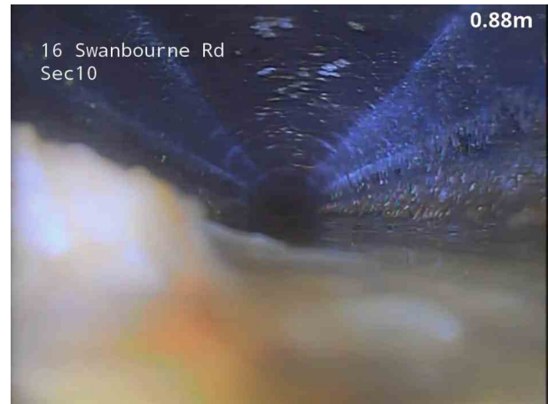
4, 00:00:11, 1.00 m Water level, 25% of the vertical dimension, Continuous
