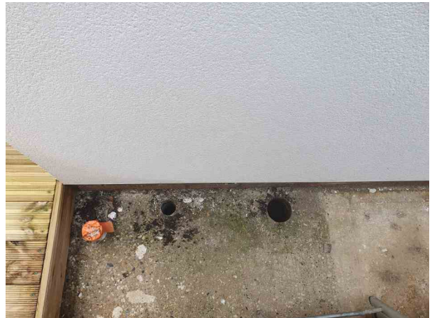
RWP and FP access
